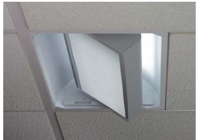
Fixture shown with 2-Lamp Rotate carriage.
